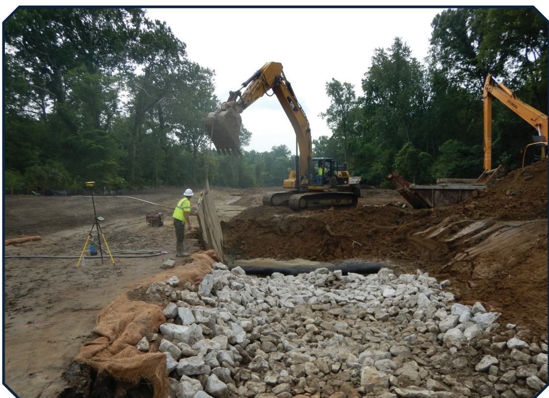
Construction of fishway.
